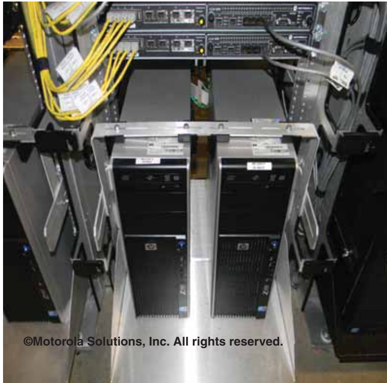
Figure 9-16 Example of Securing Equipment
