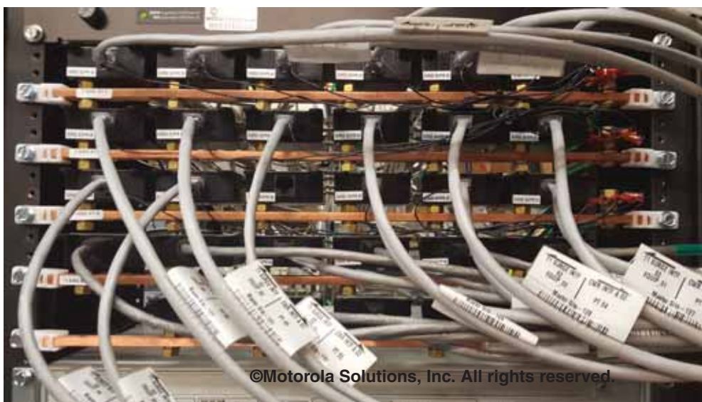
Figure 5-120 Example of Multiple Line Secondary Surge Protective Device
