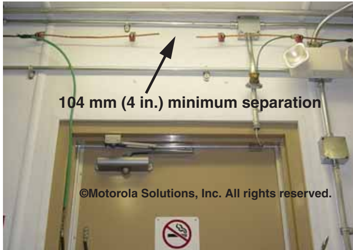
Figure 5-56 Example of Internal Perimeter Bonding Bus Conductors Separation - Opposite Primary Bonding Bar
