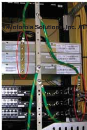
Figure 5-32 Rack with Two Network-Equipment Bonding Bars
