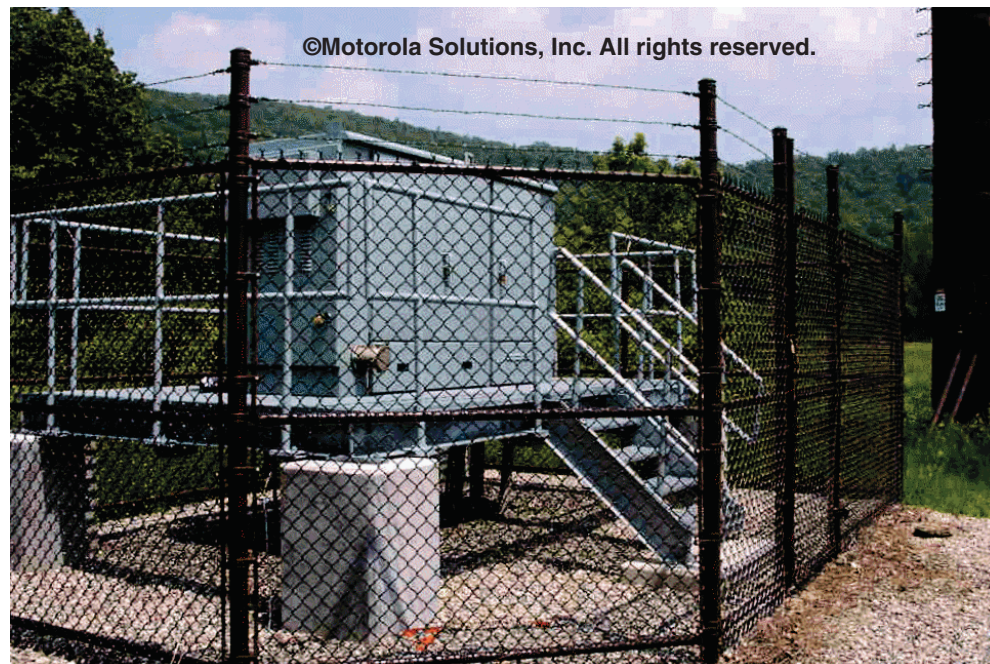
Figure 3-3 Typical Outdoor Enclosure Cabinet on Raised Platform
