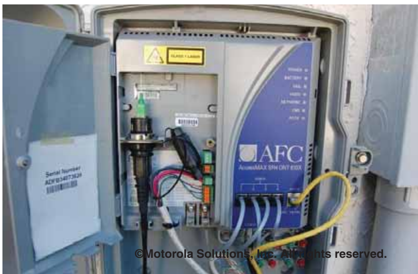
Figure 7-17 Typical Carrier Optical Network Terminal
