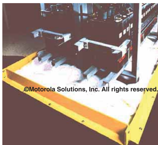
Figure 6-18 Example of Battery Spill Containment System
