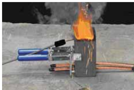
STEP 5: Reaction occurs. Wait 15-20 seconds, open mold and remove connection. Remove slag before making the next connection.
