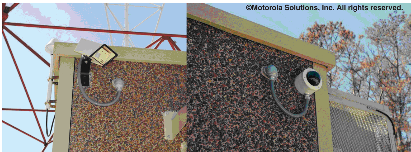
Figure 9-57 Securing and Protecting Surveillance Equipment Cabling
