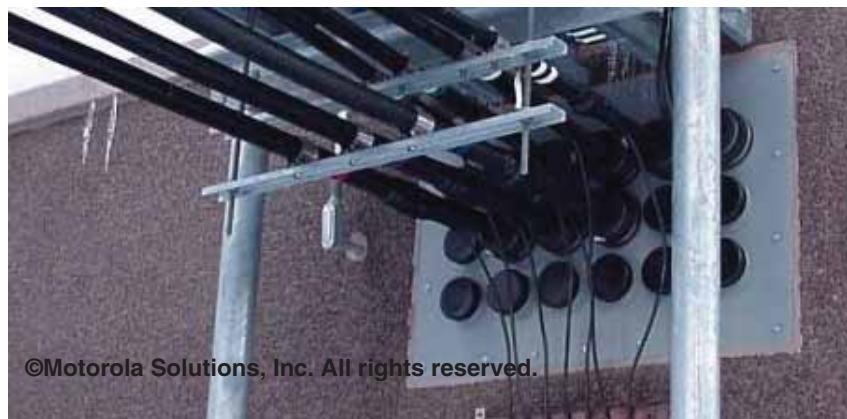
Figure 3-6 Typical Entry Plate
