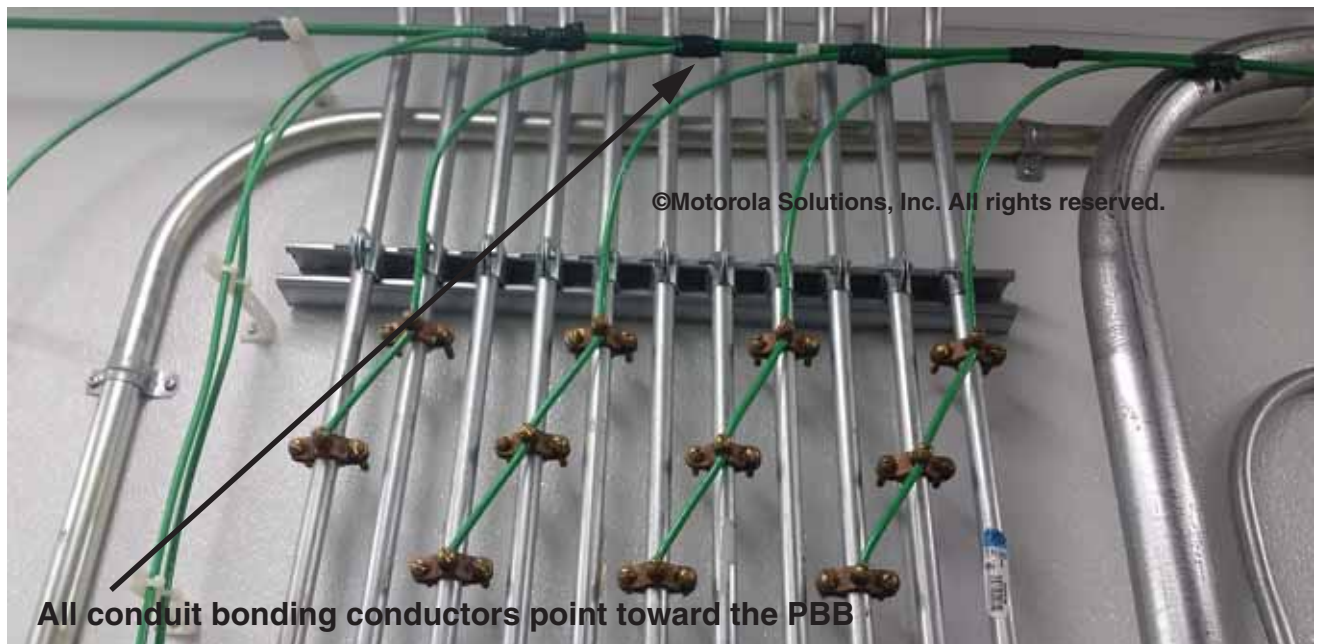
Figure 5-100 Example of Bonding Conduit to Internal Perimeter Bonding Bus
