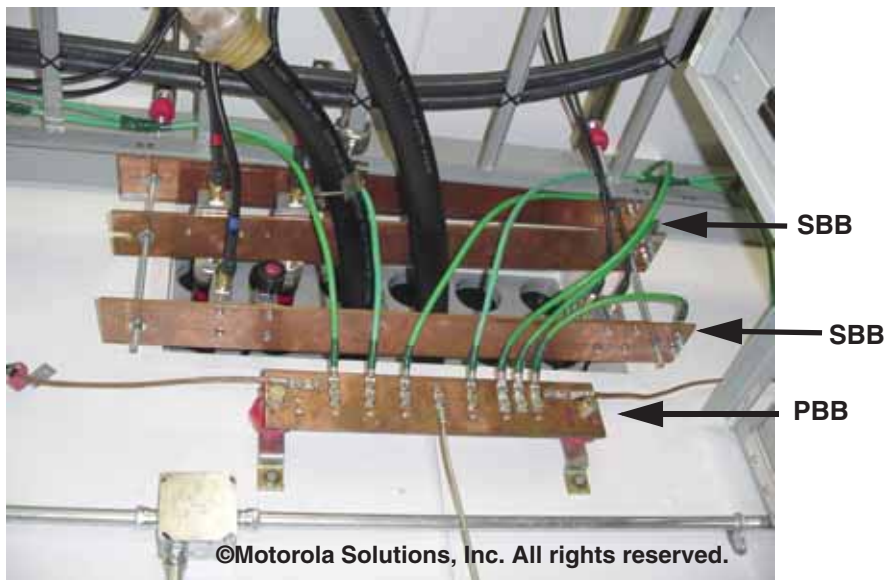
Figure 5-22 Ceiling Supported Secondary Bonding Bars at a Ceiling Level Communications Cable Entry
