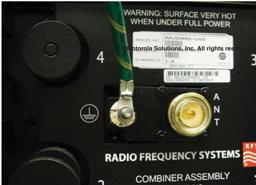
Figure 5-87 Example of Equipment Bonding - Antenna Combiner
