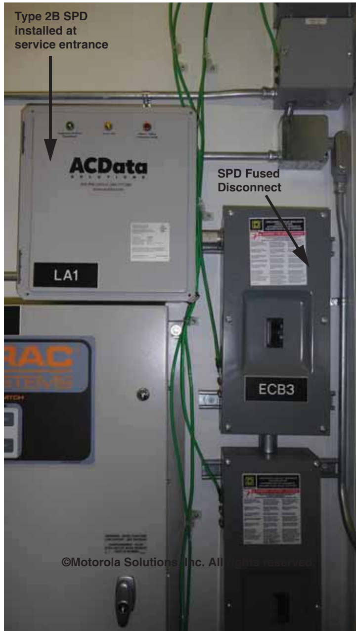
Figure 7-8 Example of Type 2B SPD Installed at Building Entry
