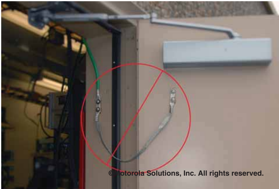
Figure 5-45 Improper Use of Flat Braided Bonding Conductor
