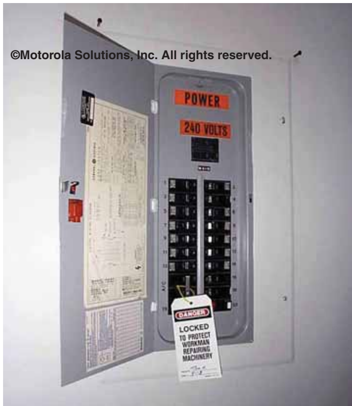
Figure 6-1 Proper Tagout of Circuit
