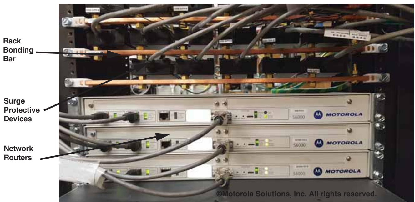
Figure 7-16 Secondary Surge Protective Devices Installed Near Protected Equipment
