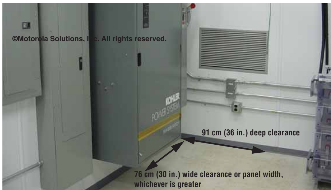
Figure 9-1 Example of Equipment Spacing
