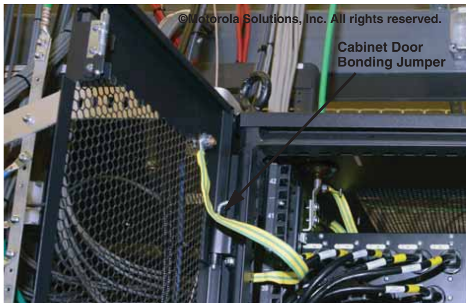
Figure 5-47 Example of Cabinet Door Bonding Jumper
