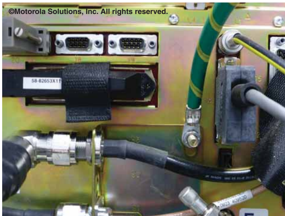
Figure 5-88 Example of Equipment Bonding - Base Station/Repeater
