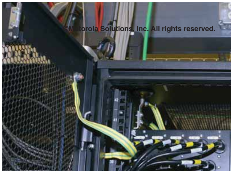
Figure 5-93 Example of Removable Cabinet Door Bonding
