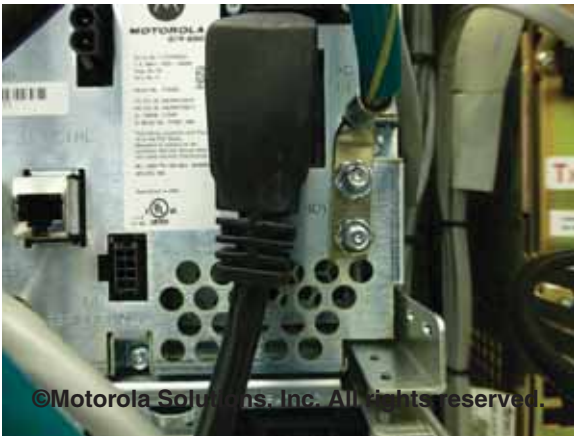
Figure 5-91 Example of Equipment Bonding - Base Station/Repeater
