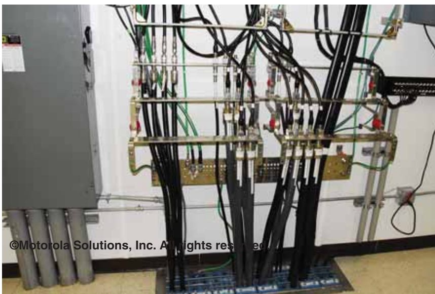
Figure 5-23 Wall Supported Secondary Bonding Bar at a Floor Level Communications Cable Entry Port
