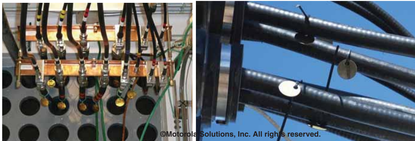
Figure 9-52 Examples of Interior and Exterior Cable Labeling
