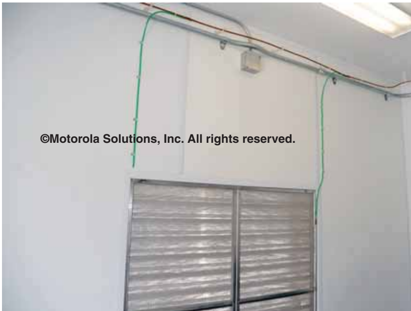
Figure 5-106 Example of Bonding Fresh Air Vent for Generator Room to Internal Perimeter Bonding Bus
