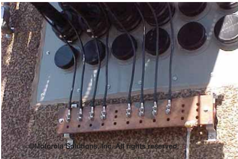
Figure 3-4 Single-Point Grounding at Entry to Building
