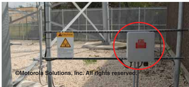
Figure 7-38 Tower Light Controller Installation
