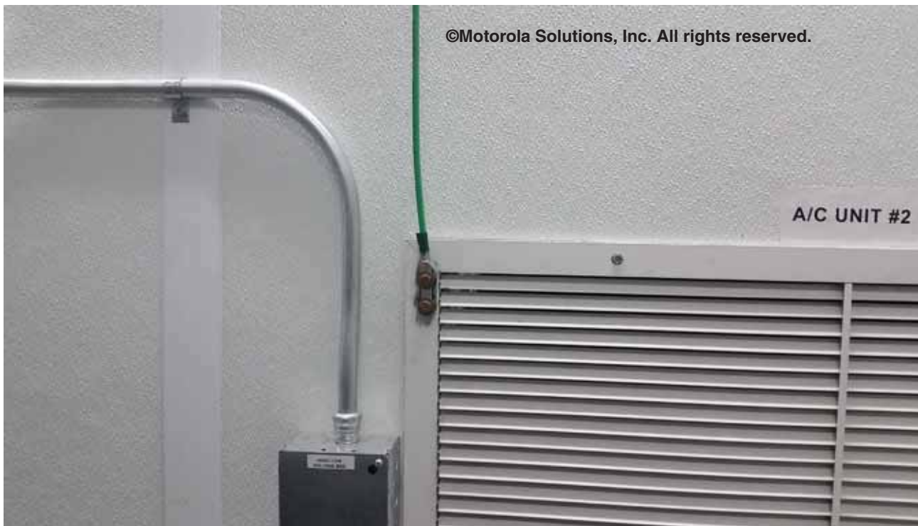
Figure 5-101 Example of HVAC Grill Bonding
