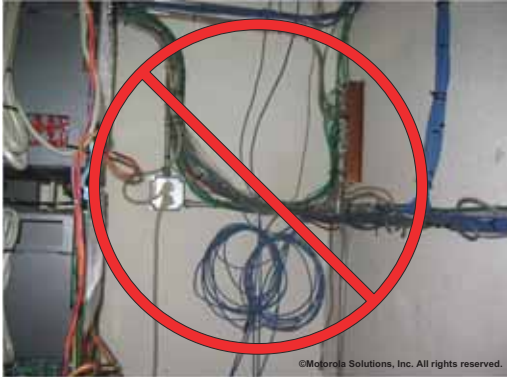
Figure 9-17 Example of Incorrectly Secured Cabling
