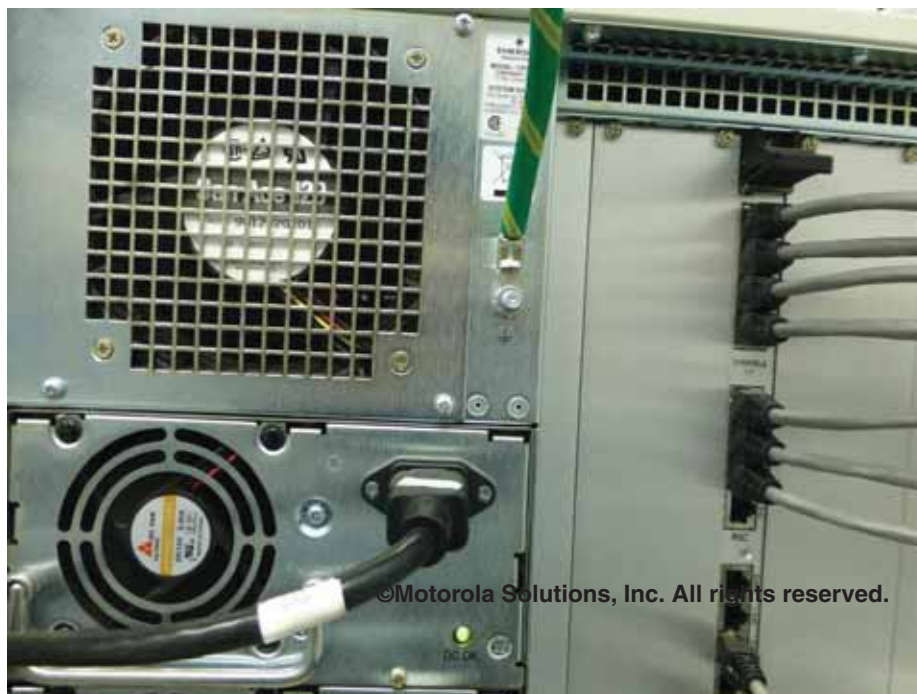
Figure 5-90 Example of Equipment Bonding - Trunking Controller
