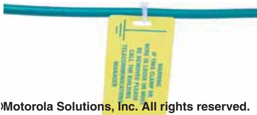
Figure 5-24 Secondary Bonding Bar Grounding Electrode Conductor Identification
