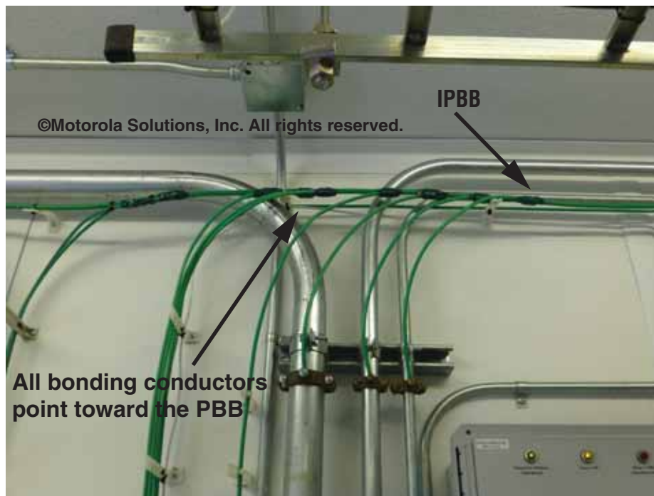
Figure 5-75 Bonding to the Internal Perimeter Bonding Bus (IPBB) Conductor
