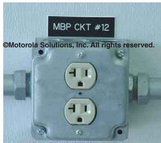
Figure 6-6 Receptacle Circuit Identification
