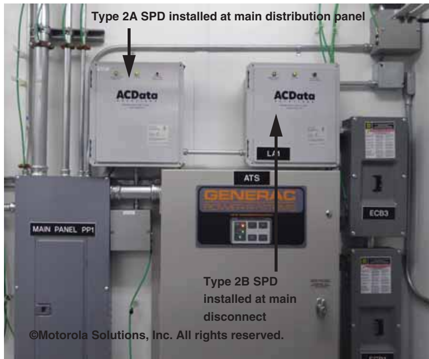
Figure 7-6 Example of AC SPD Installation at Typical Communications Site
