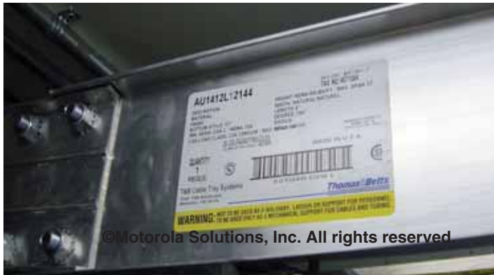
Figure 5-96 Cable Tray Listed as Equipment Grounding Conductor
