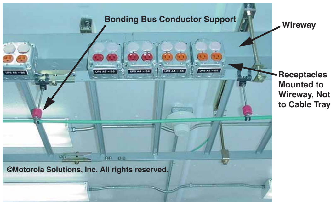
Figure 5-40 Supporting Bonding Bus Conductor on Outside of Cable Tray
