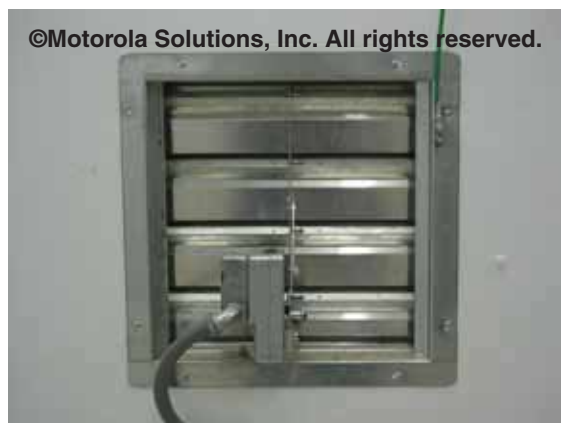
Figure 5-105 Example of Exhaust Louver Bonding
