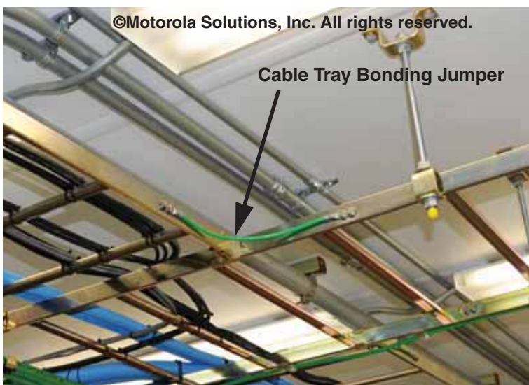
Figure 5-46 Examples of Bonding Cable Tray Sections
