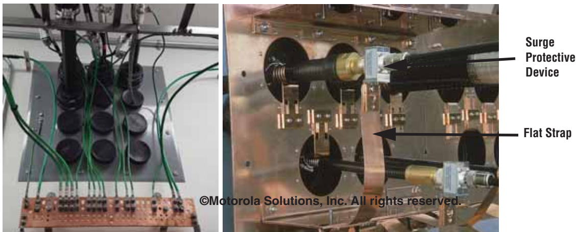
Figure 7-32 Examples of RF SPD Bonding - Round Conductor and Flat Strap (Preferred)
