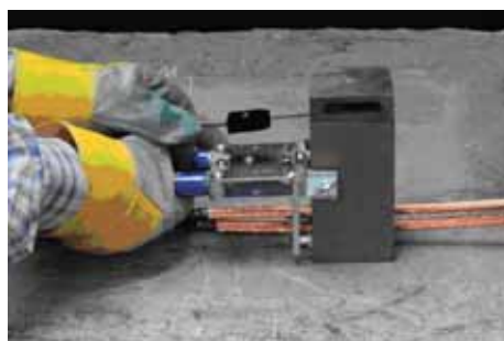
STEP 3: Attach ignition cord to the electronic igniter.
