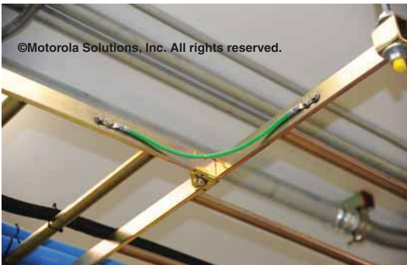
Figure 5-97 Example of Bonding Jumper Installed on Cable Tray System
