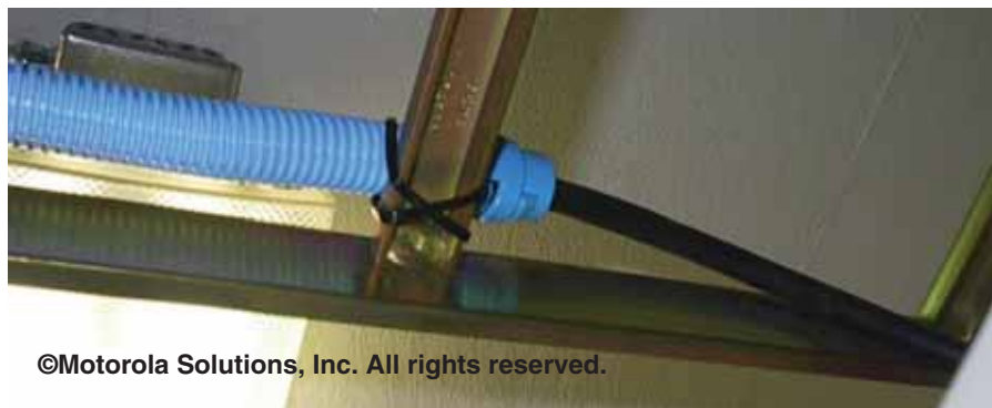
Figure 9-30 DC Power Conductor Routed in ENT
