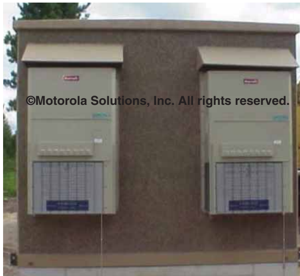
Figure 3-7 Typical Commercial Wall-Mounted Air Conditioning Unit
