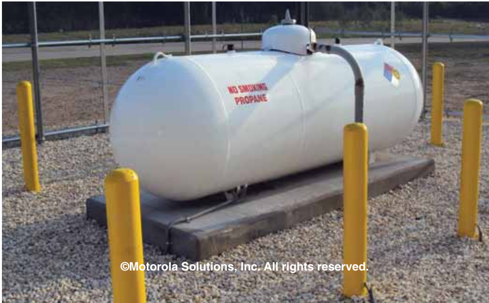
Figure 4-92 Example of Above-Ground Propane Tank Grounding
