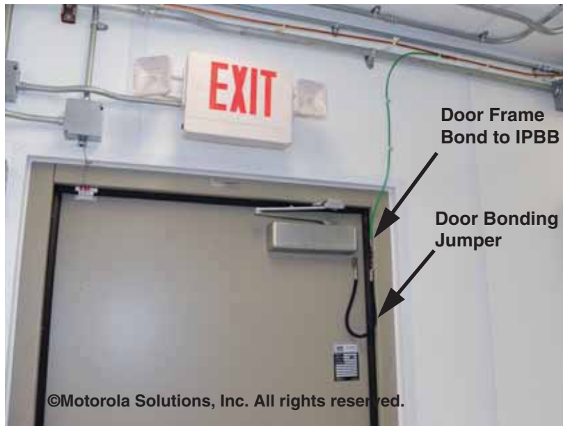
Figure 5-109 Example of Bonding Door Frame to Internal Perimeter Bonding Bus
