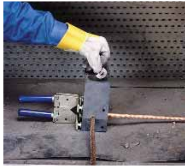
STEP 2: Close handle clamp and lock mold. Insert disk into mold.
