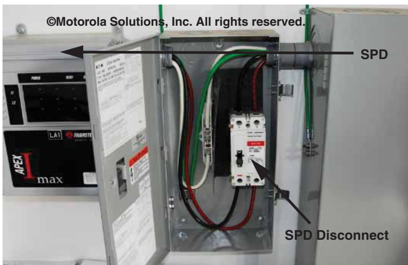
Figure 7-11 Example of SPD Exterior Disconnect
