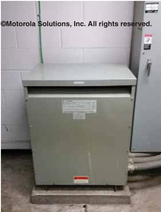
Figure 5-79 Example of Transformer
