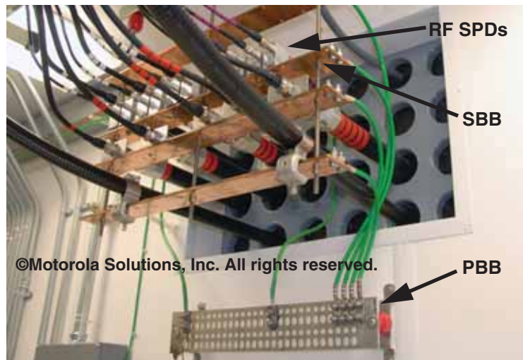
Figure 5-116 Example of RF Surge Protective Devices Bonding Directly to Secondary Bonding Bars
