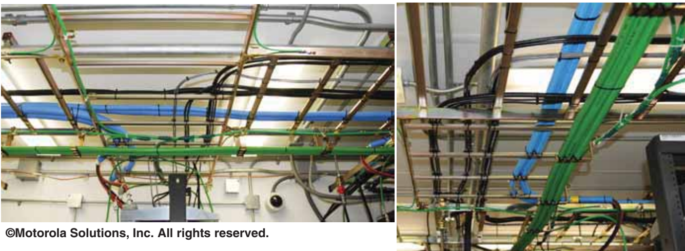
Figure 9-25 Proper Securing of Cables in Cable Tray
