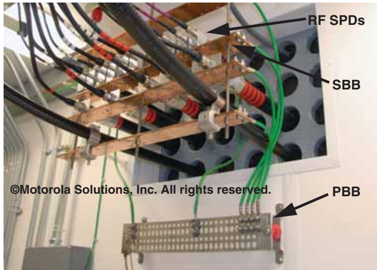
Figure 7-31 Example of RF Surge Protective Devices Bonding and Grounding Directly to Secondary Bonding Bars
