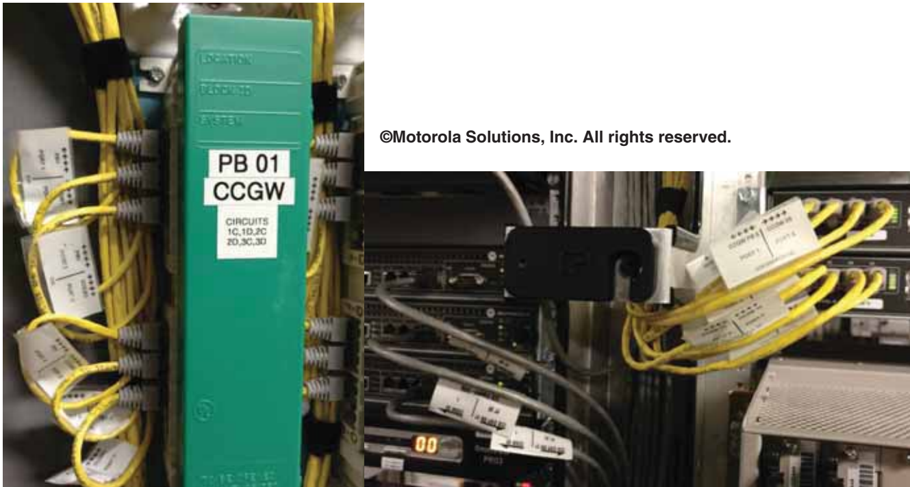
Figure 9-51 Examples of Cable Labeling
