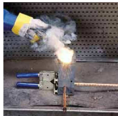
STEP 6: Wait 15 to 20 seconds for the reaction to complete, then open the mold and remove the welded connection. Remove slag from the mold before making the next connection.
