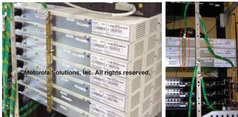
Figure 5-33 Typical Network-Equipment Bonding Bar Mounting Locations
