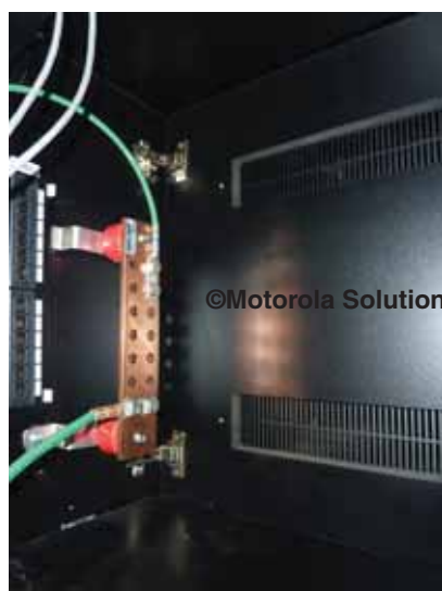
Figure 5-138 Example of Secondary Bonding Bar at Operator Position
