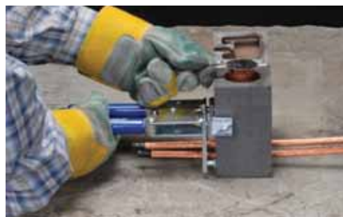
STEP 2: Close and lock handle clamp. Insert drop-in cartridge into mold.
