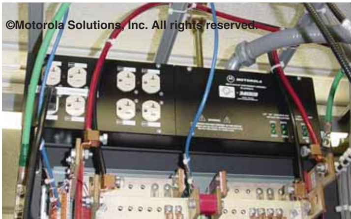
Figure 9-28 Example of Rack Mounted Receptacle Assembly
